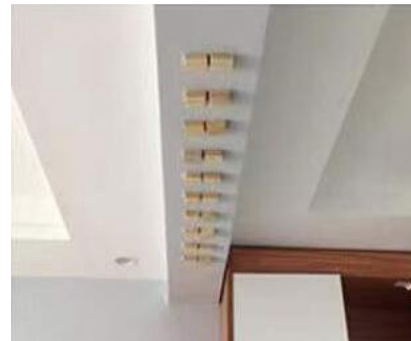
1. Fix the wood blocks in equal distance on the top.
