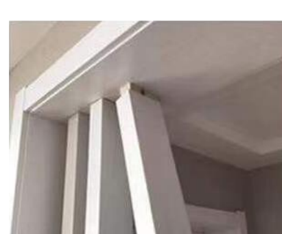
3. Fixing the tube and wood blocks on the top.
