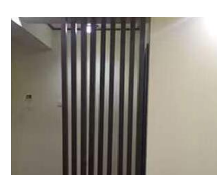
4. Finishing Tube Installation.
